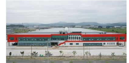
산업설비 (Industrial Facility)
