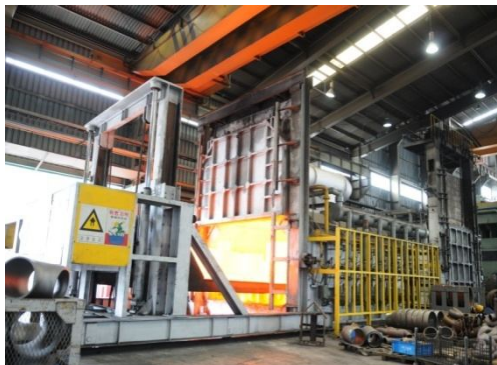
Heat Treatment Furnace For Fitting
