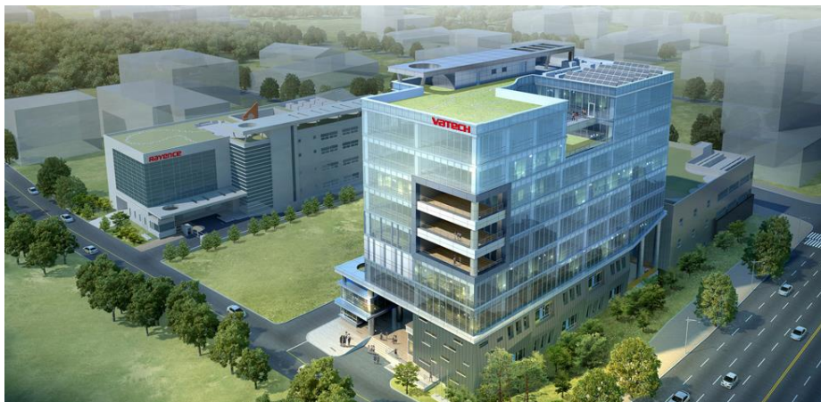
Buildings view in Dong-tan area, Gyeonggi province
